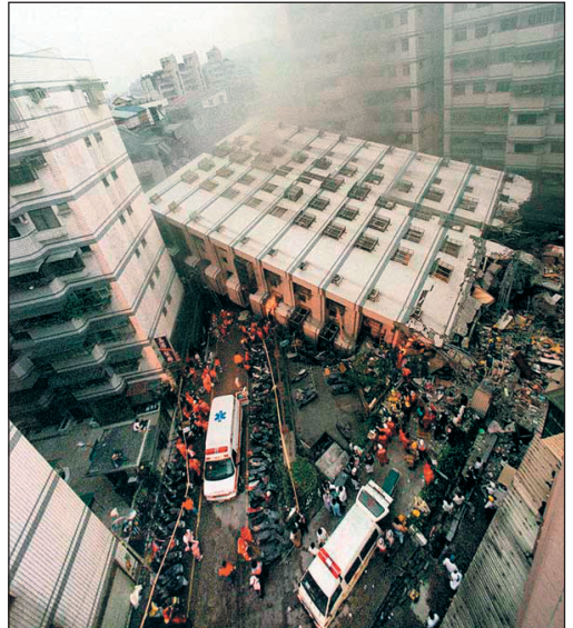
Taiwan apartment block toppled by 1999 quake
